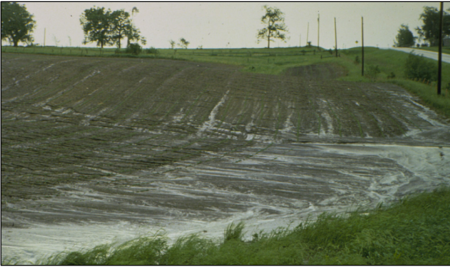
Signs of Erosion – Small rills and channels on the soil surface are a sign of water erosion
